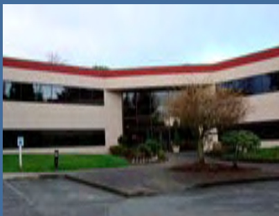
Federal Way, Seattle (USA) home to the technical services team, and a world-class data centre.
